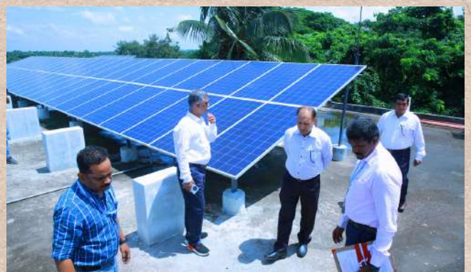
Visit to Solar System Facility
